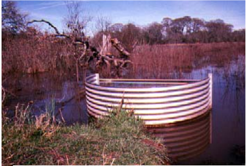
A flashboard riser box attaches to a pipe installed in a levee to create a shallow water wetland for wildlife.
