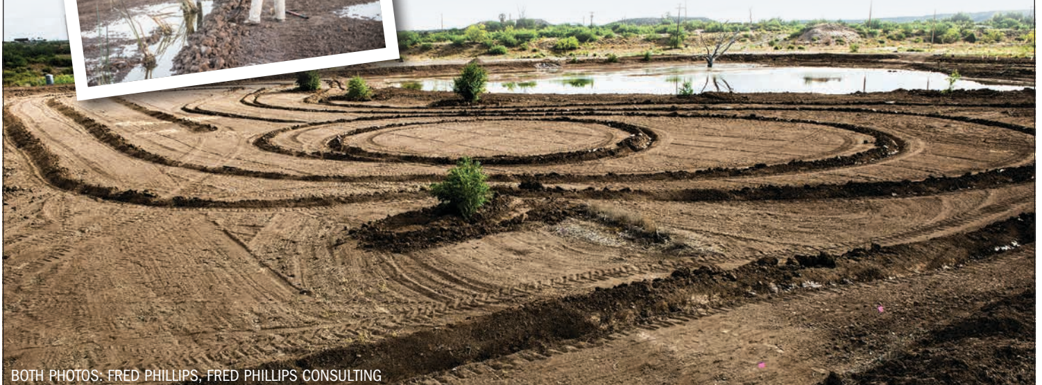
Furrow ditches made with a tractor made for easier and more efficient planting of the wetland plugs.
