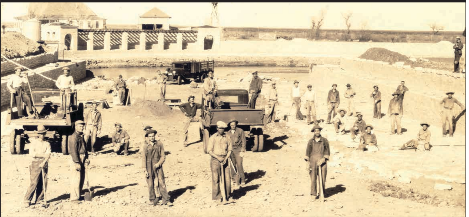
Civilian Conservation Corps workers build the swimming pool at Balmorhea State Park.
