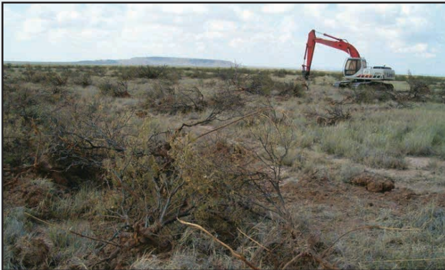
Excavator grubbing western honey mesquite. Photo provided by Bonnie Warnock, Sul Ross University.
