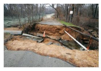
Figure 7.8 - Floods in Bastrop followed the fires. Rain soaked soils laid bare by the fire quickly eroded and washed out waterways. Here the earthen dam was washed out on Copperas Creek, draining the lake in Bastrop State Park. Image courtesy of TPWD.
