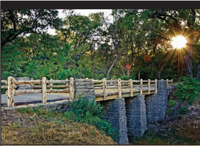
Camp Creek Bridge, built by the Civilian Conservation Corps, is easy to see from the scenic park road.
