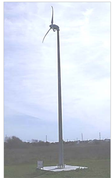
A 3kW wind turbine provided by the Galveston Island State Park Friends Group.
