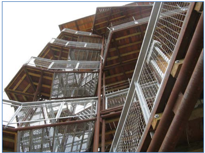
The use of reclaimed surplus oil field pipe at the Sheldon Learning Center Observation Tower is located in an industrial area, east of Houston, an area known for oil production.
