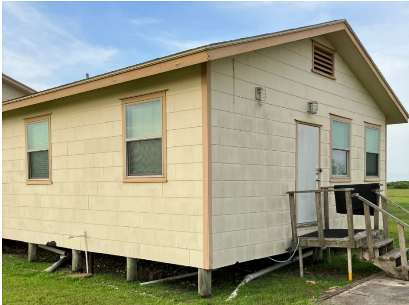
4. Bunkhouse. Attic wall vent shown.
