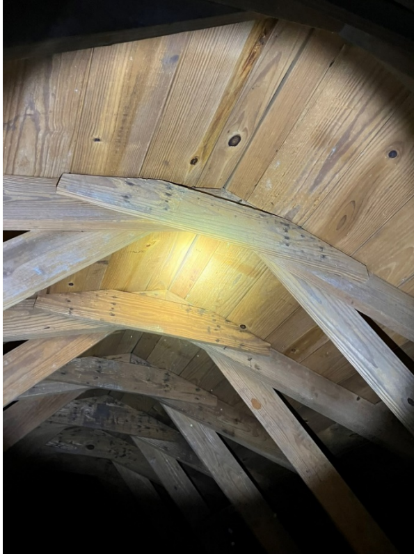
7. Bunkhouse: Truss and decking shown from inside attic.
