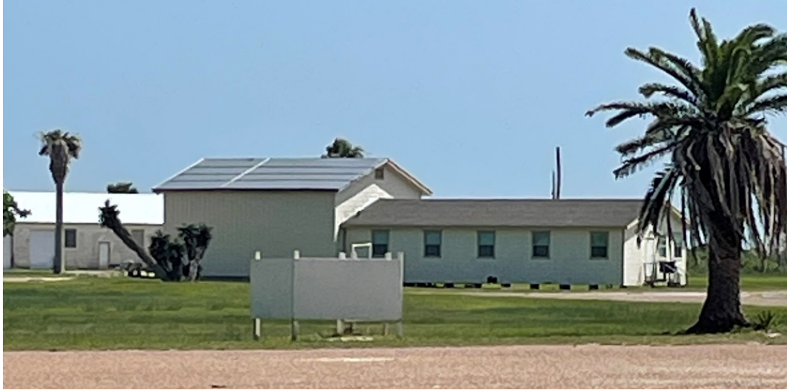
1. Bunkhouse/Garage. Garage roof is tarped. White roof in background is not in contract.
