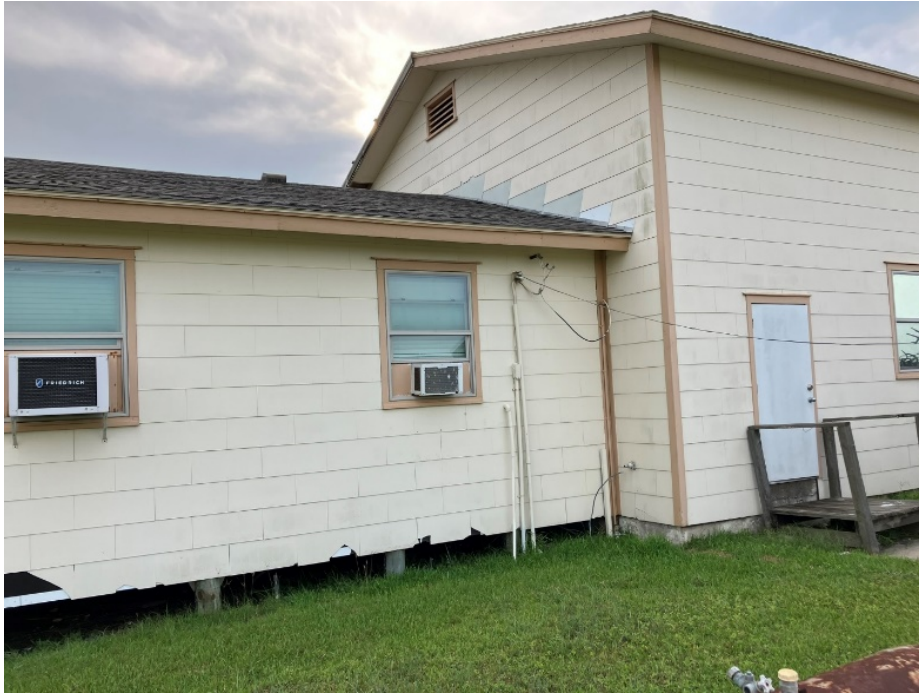
5. Bunkhouse/Garage. Note the sidewall flashing at Garage.
