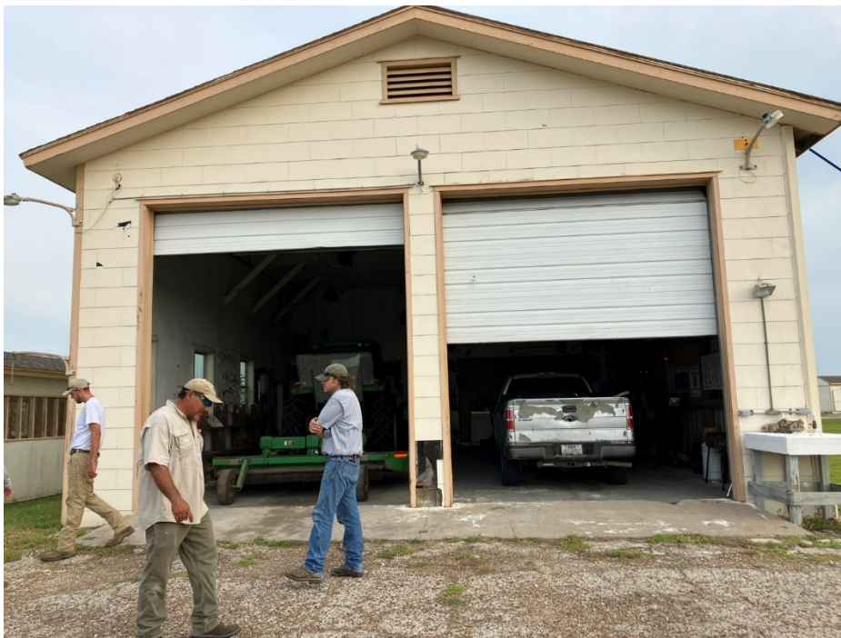
6. Garage. Garage attic wall vent shown. Adjacent shed partially shown.
