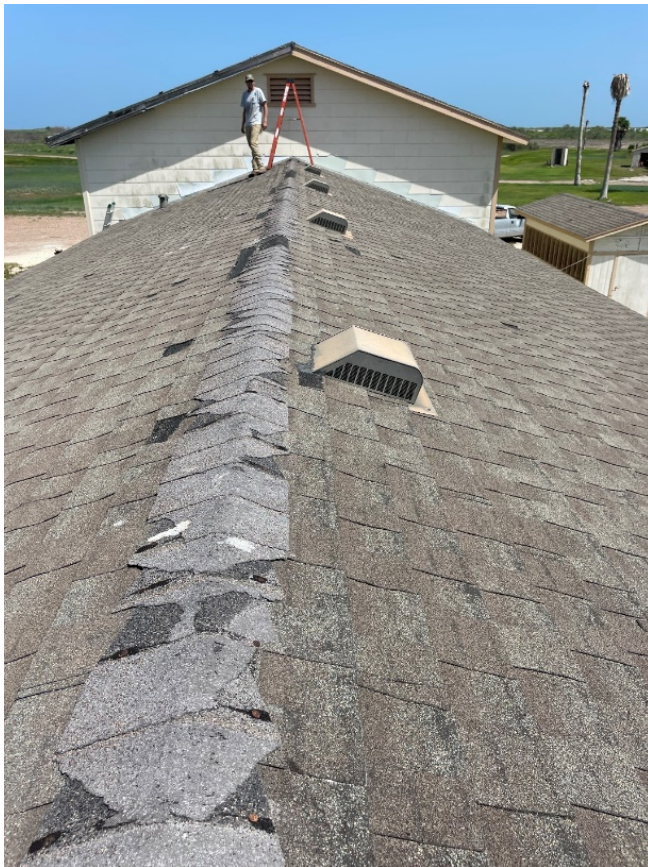
2. On top of Bunkhouse. Note the sidewall flashing at Garage wall.
