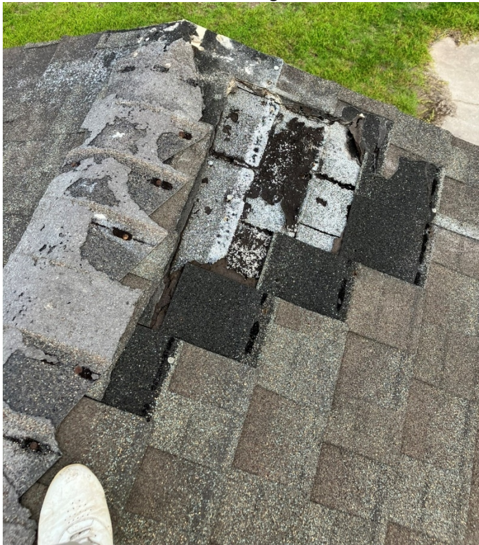
8. Bunkhouse: Composition shingles and underlayment over earlier shingles.
