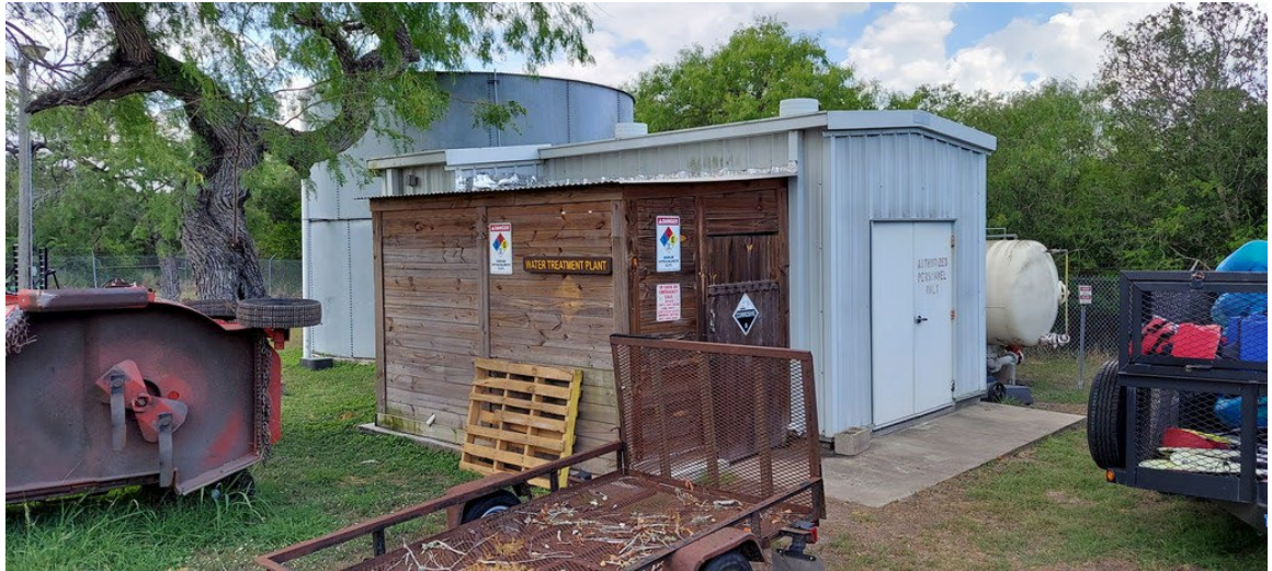
Existing Water Treatment Plant Building w/ Wooden Chlorination Shed
