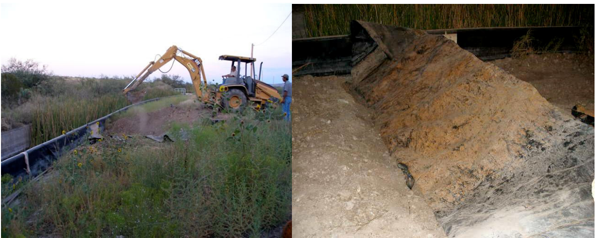
Fig. 7a & b– construction of refugium canal berm
