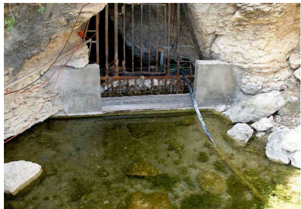
Fig. 5b –installed stop-log gate
