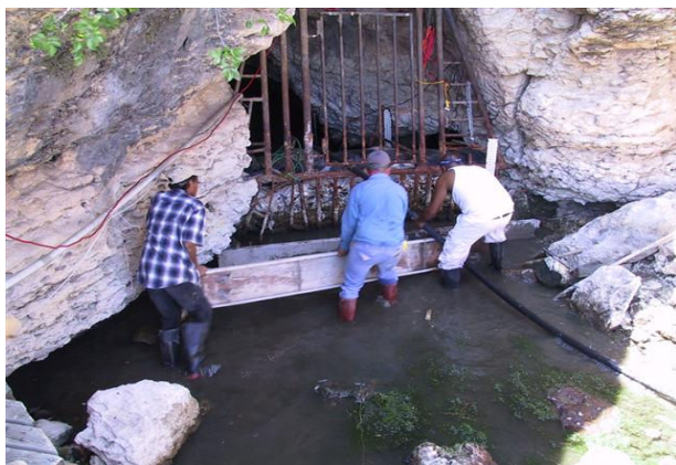
Fig. 5a – installing concrete forms
