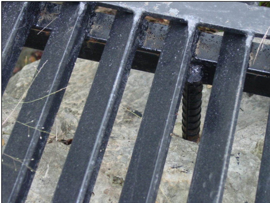
Figure 2-8. Example of Anchor Rebar
