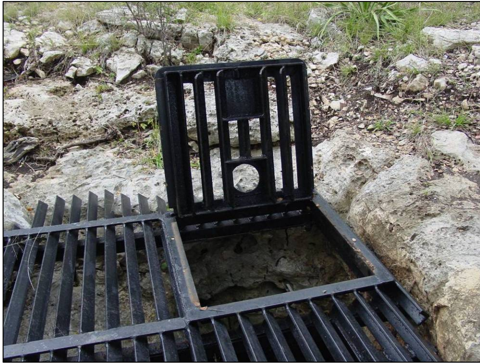
Figure 2-9. Example Cave Gate Access
