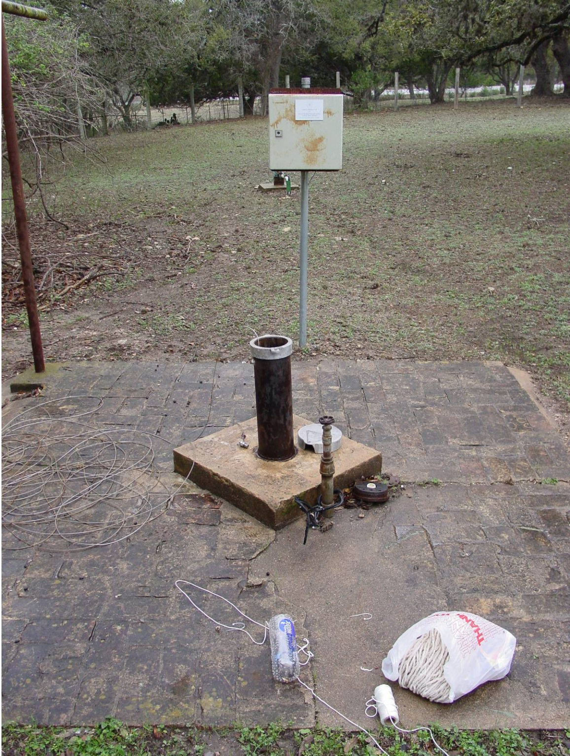
Figure 6. Dowell Well (TWDB ID # 58-50-801) located just north of Onion Creek in Manchaca, Texas. Note bottle trap and mop head in foreground.
