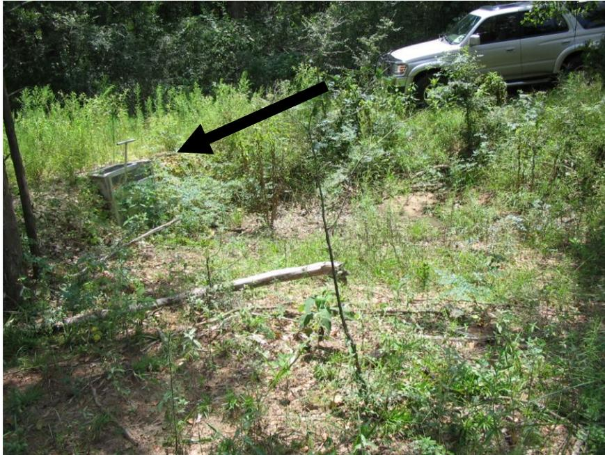
Ephemeral pond that was constructed in HTMA5. Arrow indicates flash-board riser, which controls water level. Pond has held water for short periods as indicated by growth of sedges, rushes and other water-loving plants.
