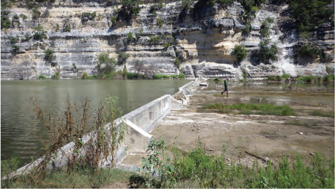
Figure 12. Dam removed from the North Fork Guadalupe River to restore instream connectivity and fish passage.
