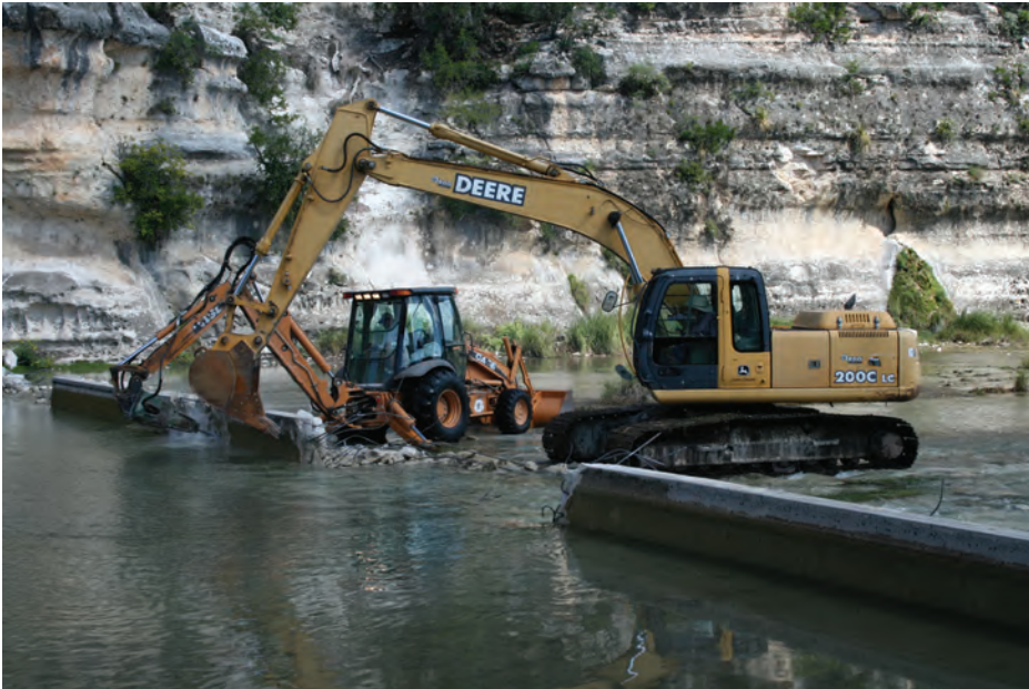
Figure 13. Active removal of a dam on the North Fork Guadalupe River to restore instream connectivity and fish passage.
