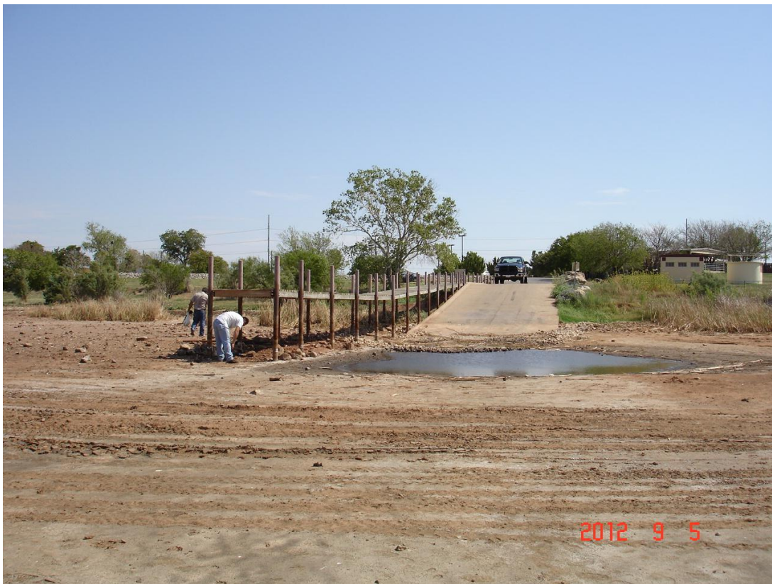
Figure 4. Photograph of the Lake Wichita boat ramp.
