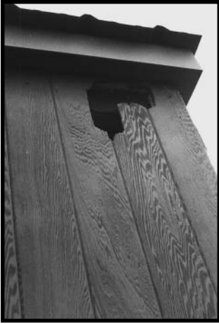
This L-shaped hole was large enough for a large raccoon to enter.
