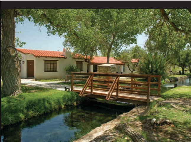
A canal flows past the San Solomon Courts.
