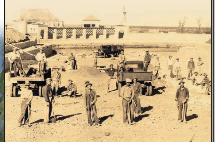
CCC Company 1856 builds the pool around San Solomon Springs.
