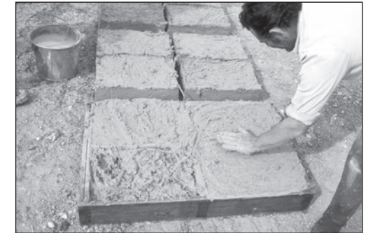
Adobe brick making during restoration
