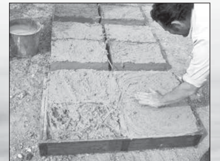
Adobe brick being made during restoration work.
