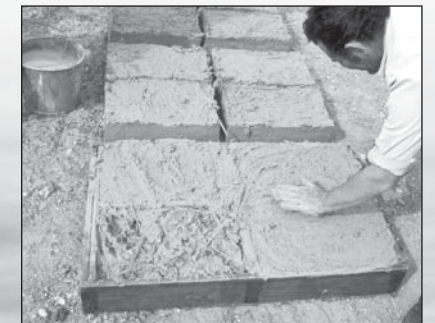
Adobe brick being made during restoration work.
