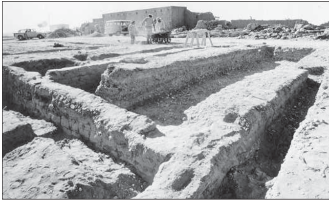
Fort Leaton in 1971 during archeological investigations and restoration work
