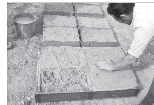
Adobe brick making during restoration
