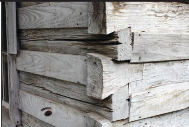
The second and third rooms were constructed of logs hewn on both sides and joined at the corner with half dove-tail notching. This is considered the best technique for building log homes.
