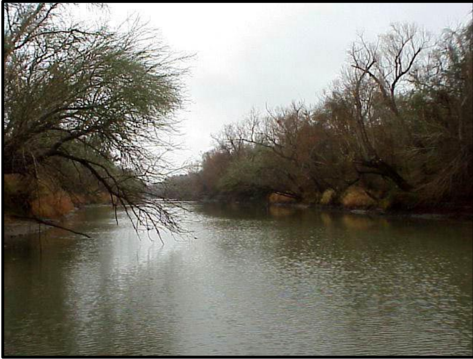
Figure 4 Nueces River at US 59 bridge near George West, Texas.
